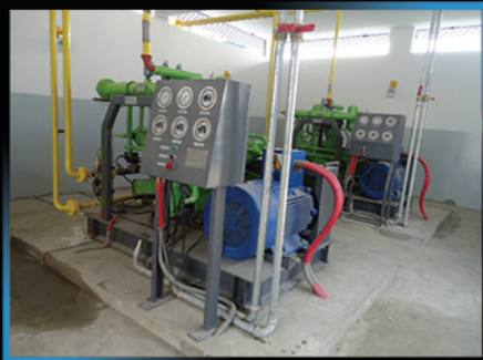
Al-Riaz International CNG Station, Rawat (Islamabad)
