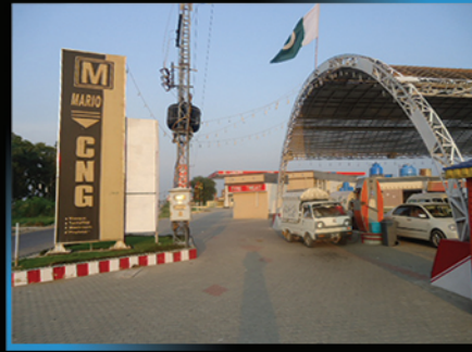
Mario CNG Station, Sara-e-Alamgir
